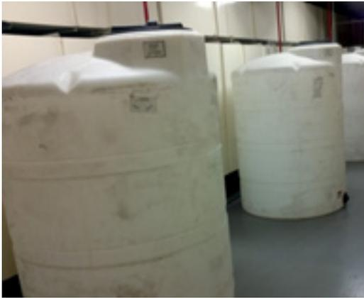
Two roof drains are projected to divert 68,000 gallons of rainwater per year into seven, five-hundred gallon tanks. The tanks can store up to 3,500 gallons of rainwater.
